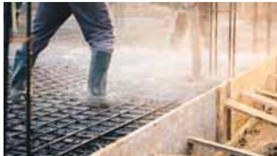
(b): In-situ cast concrete for a road bridge
