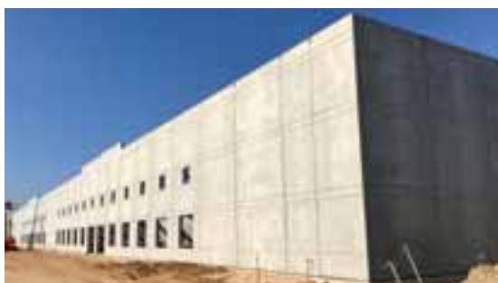
(c): Pre-cast concrete elements for a multi-storey dwelling
