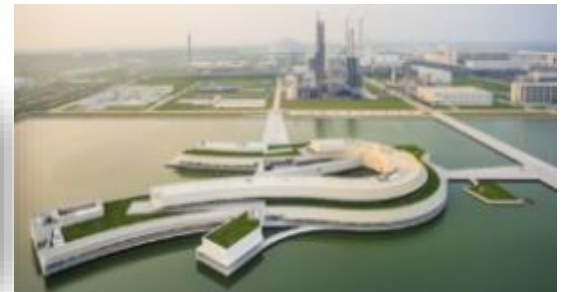
7. Cast in-situ concrete: Huai'an Shilian Chemical Plant, China | Architect: Alvaro Siza
