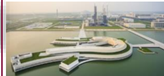
8. Cast in-situ concrete: Huai'an Shilian Chemical Plant, China | Architect: Alvaro Siza
