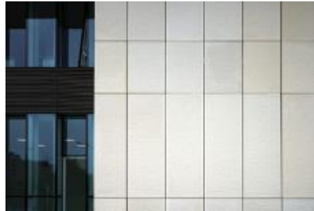
1. Pre-stressed concrete façade: Chengdu Jingchuan Office Building, China
