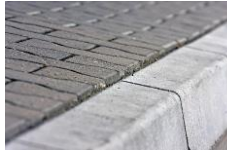
2. Paving blocks: Kerb, Poland
