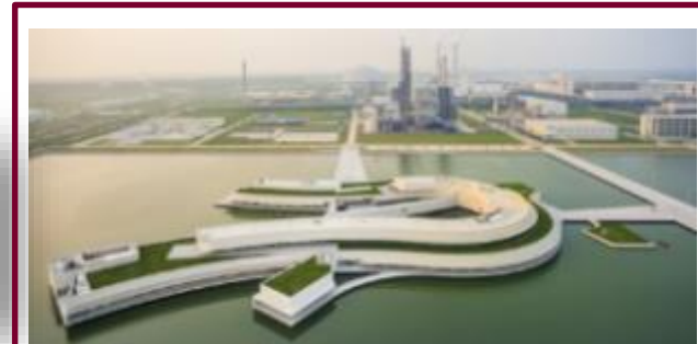
7. Cast in-situ concrete: Huai'an Shilian Chemical Plant, China | Architect: Alvaro Siza
