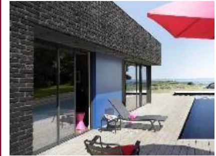
3. Artificial stone: Villa façade application, France
