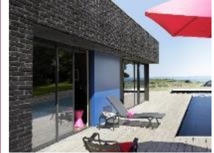
3. Artificial stone: Villa façade application, France
