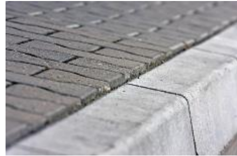
2. Paving blocks: Kerb, Poland
