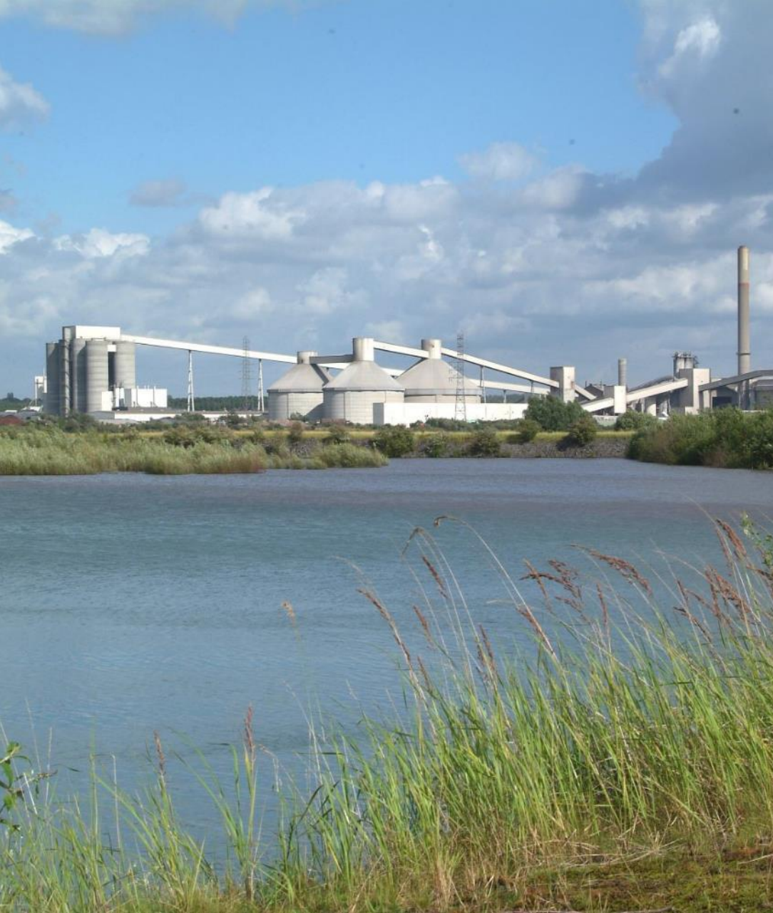
Gaurain Plant, Belgium
